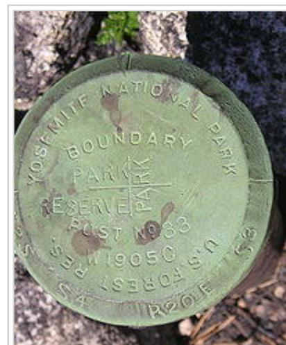
Figure 3. The engraved cap on a corner monument pipe, in western Yosemite National Park, placed in 1905 during the Park boundary resurvey
